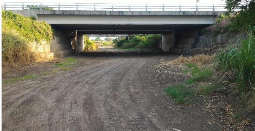
Figure 6.6: Evidence of Channelling in the Bower's Gully north of Whim Estates
